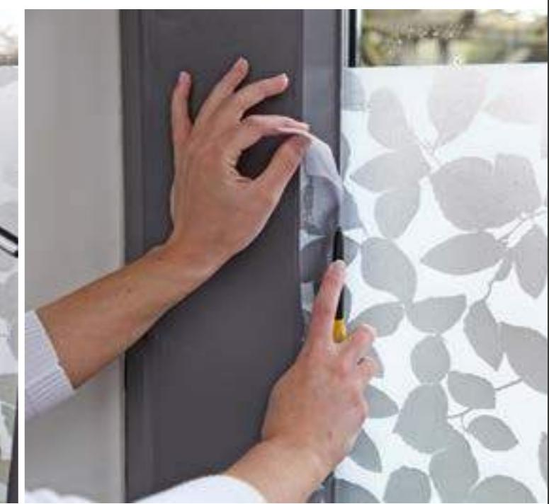
Remove excess film using a sharp knife along a ruler or straight edge, and then smooth over.
