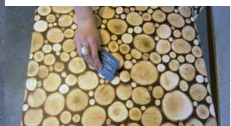
Use a wiper to smooth out the film starting in the middle in order to remove air and moisture from in between the surface and the film.
