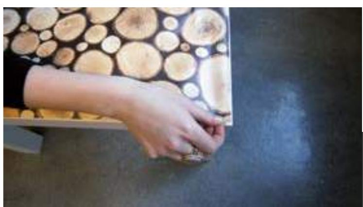
Apply the film to the surface of the section to be applied, making sure to position it carefully.
