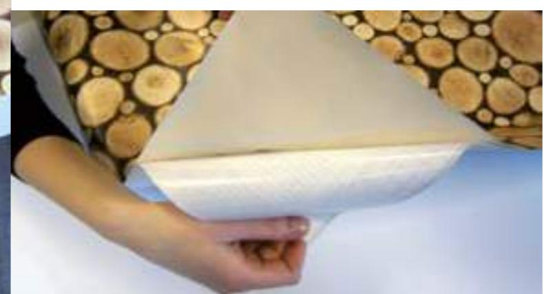
Peel the protective layer of the film. It may help to spray the surface to be covered with water.
