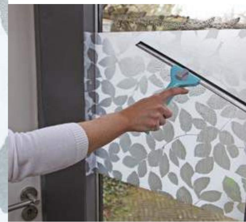
Use a window wiper to smooth out the film starting in the middle in order to remove air and moisture from in between the window and the film.
