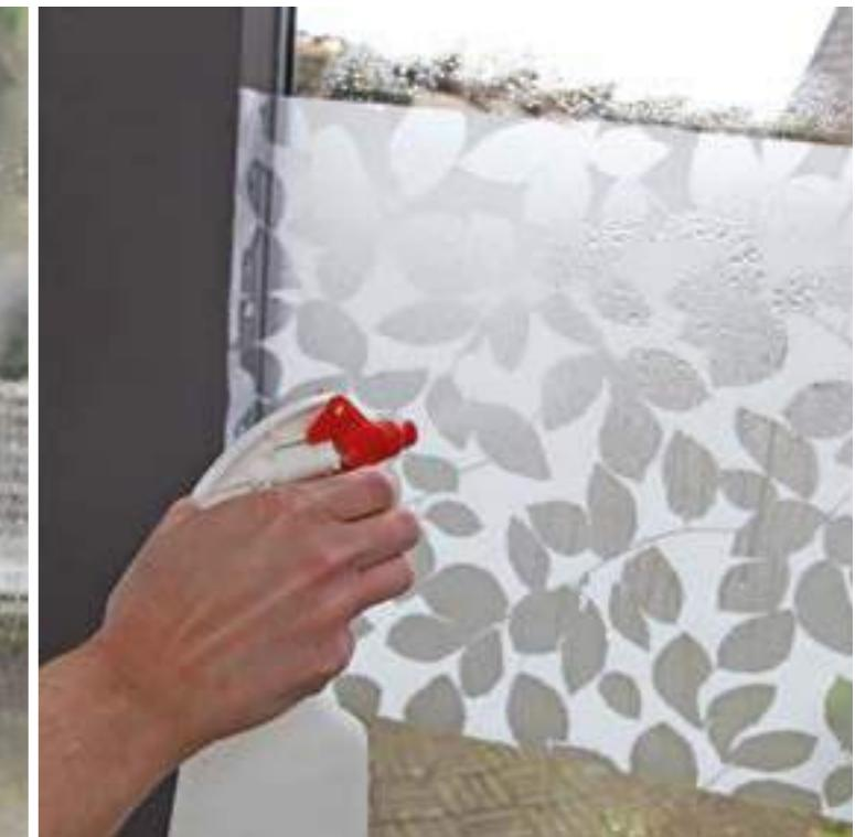
Apply the film to the window, making sure to position it carefully. Wet the outer surface of the film to prevent scratching.
