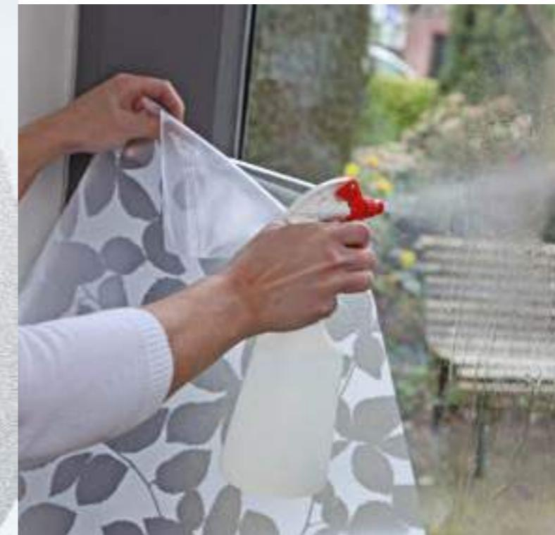
Carefully clean the surface of the section to be applied, making sure it is dust-free and smooth. Cut the film to a slightly larger size than the area to be covered. Spray the window with water. Peel the protective layer off the film.
